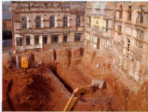
Bulk Excavation
